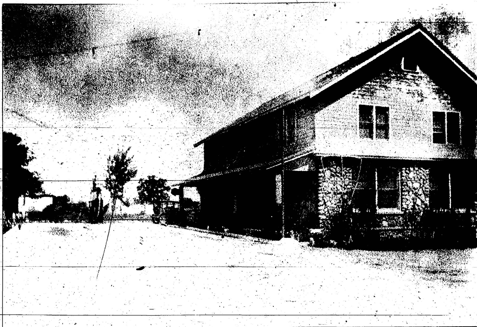
The old Pierce property on the northeast corner of M-52 and Old US-12 has been torn down to make way for a new pharmacy. Built in the late 1920s, the place served as a gas station and small diner.
